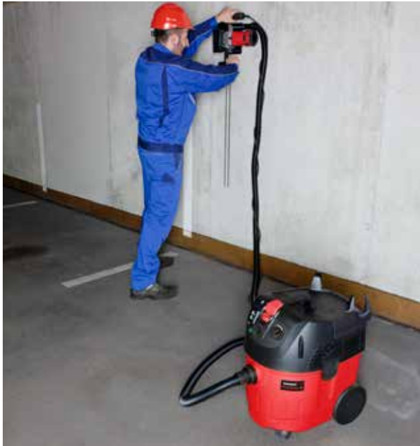
Extraction of health hazardous dusts when chasing and cutting
